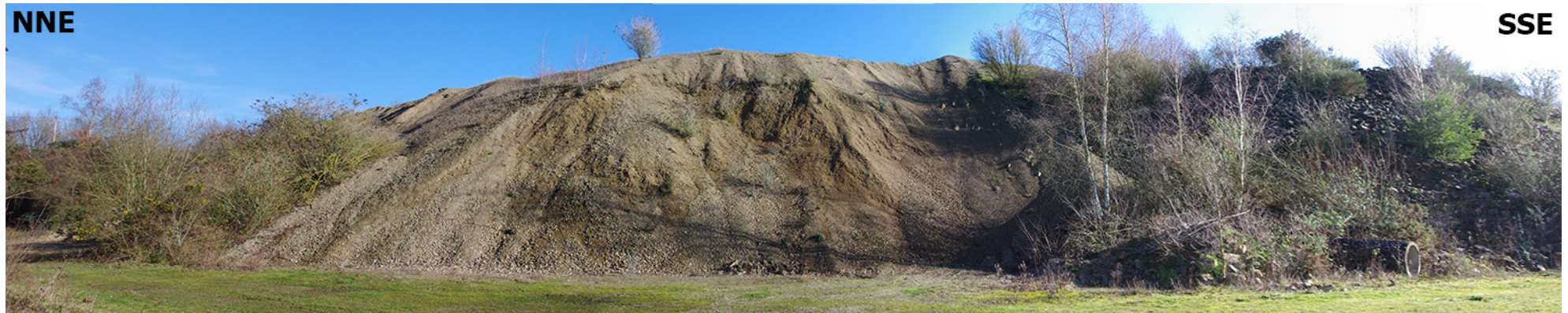
Illustration 5: Vue 5 Stockage Nord
